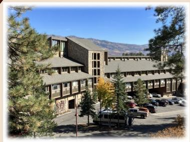
The Lodge roof was completed last November, using 30-year architectural shingles with a Class 4 impact resistant rating. This means the shingles can withstand 2" hail without sustaining serious damage. In addition, a hot edge system along with heated gutters and downspouts should minimize any icicle buildup, making the west side of the Lodge a much safer area.
