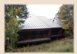
Highpoint, Pinecone, and Gamble Oak are being roofed with a 24-gauge standing seam metal roof. The concealed fastener design means that this roof requires no maintenance. Highpoint was completed earlier this year. Pinecone will be complete as of October 25th, with snow bars installed on units over the undercover parking area. By the time the snow flies, Gamble Oak should be about 40% complete.
